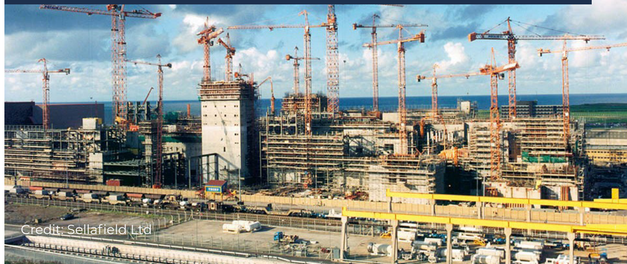
THORP: Construction of the Thermal Oxide Reprocessing Plant gets underway
