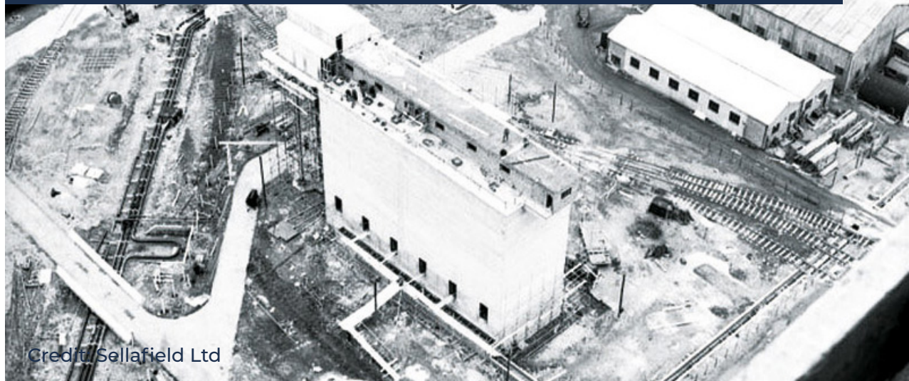
MSSS: Magnox Swarf Storage Silo begins construction
